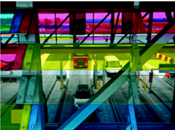
Motorway Toll, Autoroute
